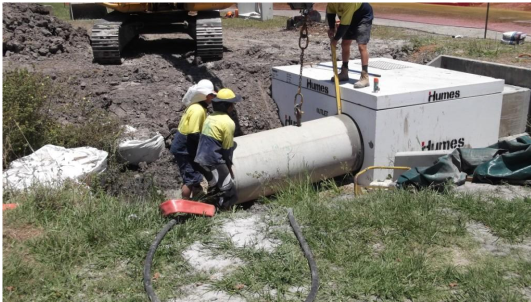
Figure 1 – Humegard® HG27 Installation at USC
